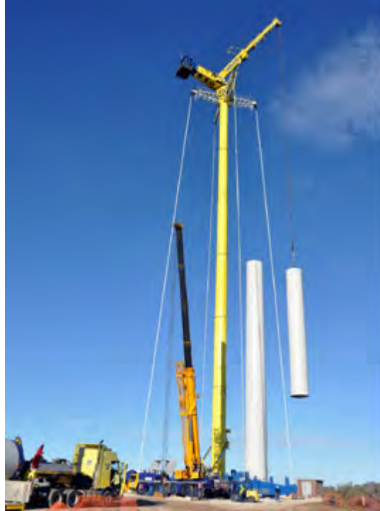
Figure 2-6: Example - Cranes at work
